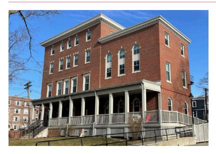
The Modernization of 116 Norfolk will preserve the historic architecture of the main convent building, the four-story wing facing Norfolk, and replace the three-story East Wing with a new addition over the existing parking lot on Suffolk Street. The porch will be partially preserved.
